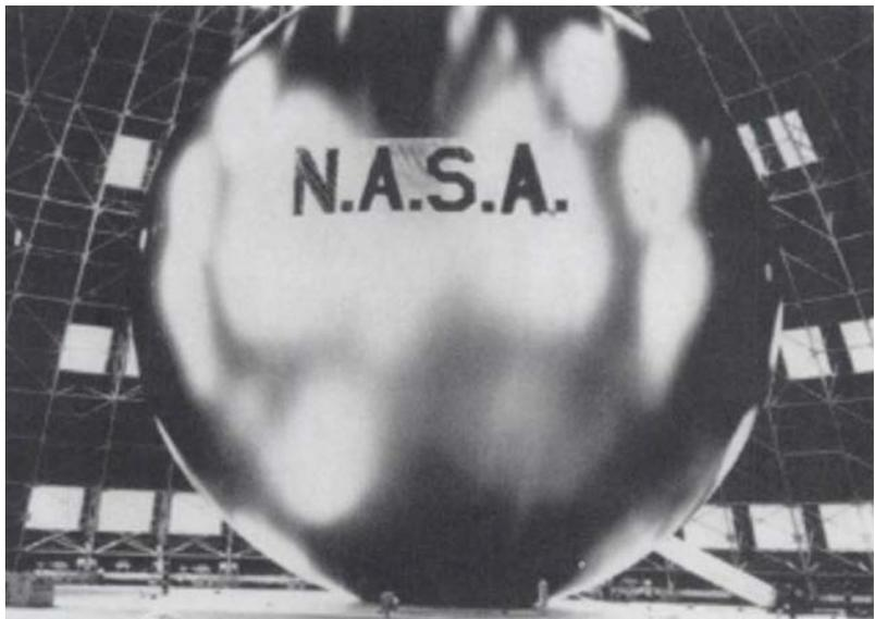
Complex membrane structures were flown in space 55 years ago and developed for terrestrial application 60 years ago. These structures massed 17.8 grams per square meter of surface area using 12-micron thick aluminum-coated off-the-shelf material. Today, 3.6-micron thick materials fabricated at a GBO film achieve 4.0 grams per square meter and less with improved optical and mechanical performance.
